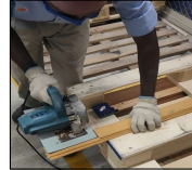
Cutting of collected angle board into required std. dimensions New angle board cost – EUR 0.2 Rework angle board cost – NIL
